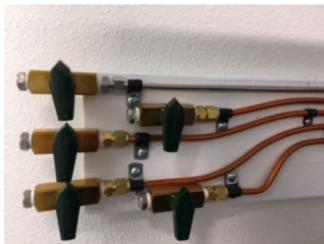
11. If the tank change takes place in the middle of the day, skip the leak check. Open the gas line valves for the gas replaced.
