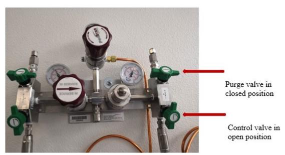
3. For the gases with no backup cylinder inlet, which are Helium + Oxygen, Helium + Methane, and Hydrogen, put the carbon analyzers on "Standby" mode before any of these gas tanks need to be changed.
